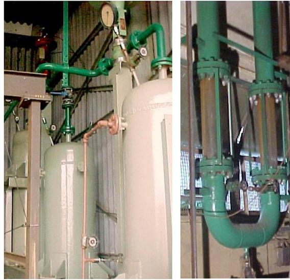
**Test Facility for Passive Containment Isolation system**
