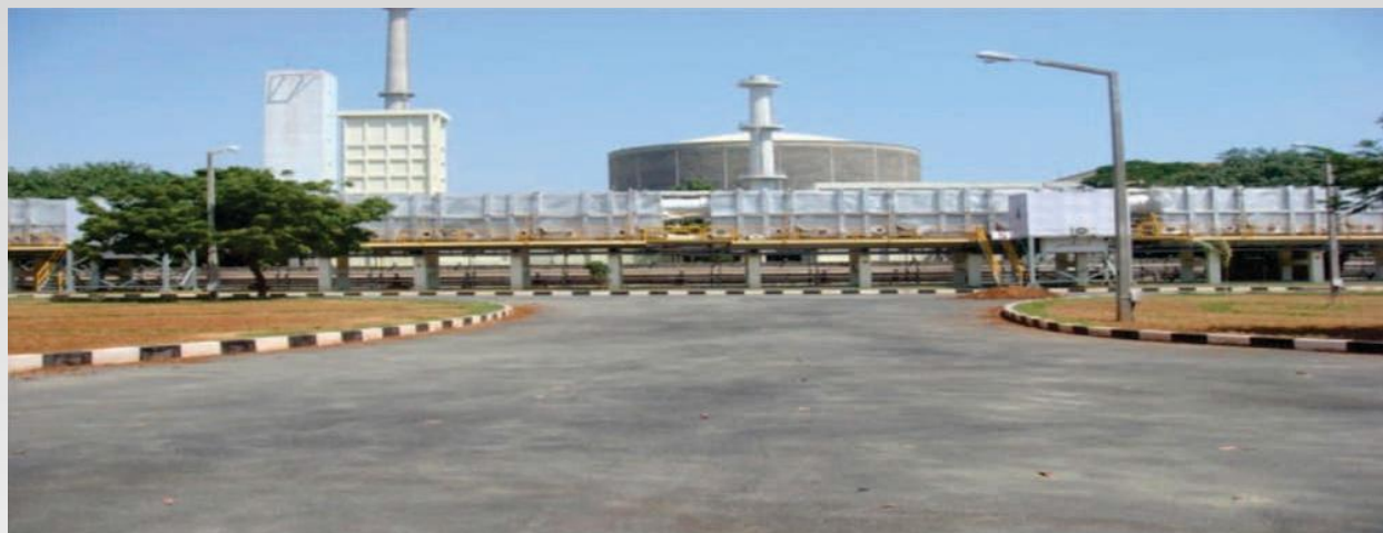
4.5 MLD Multi Stage Flash Plant at Nuclear Desalination Demonstration Plant (NDDP), Kalpakkam coupled to Madras Atomic Power Station
