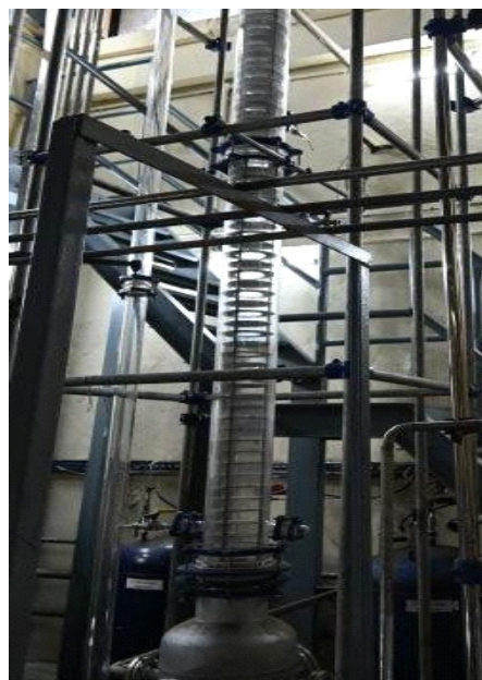
6" diameter PDDC facility.
