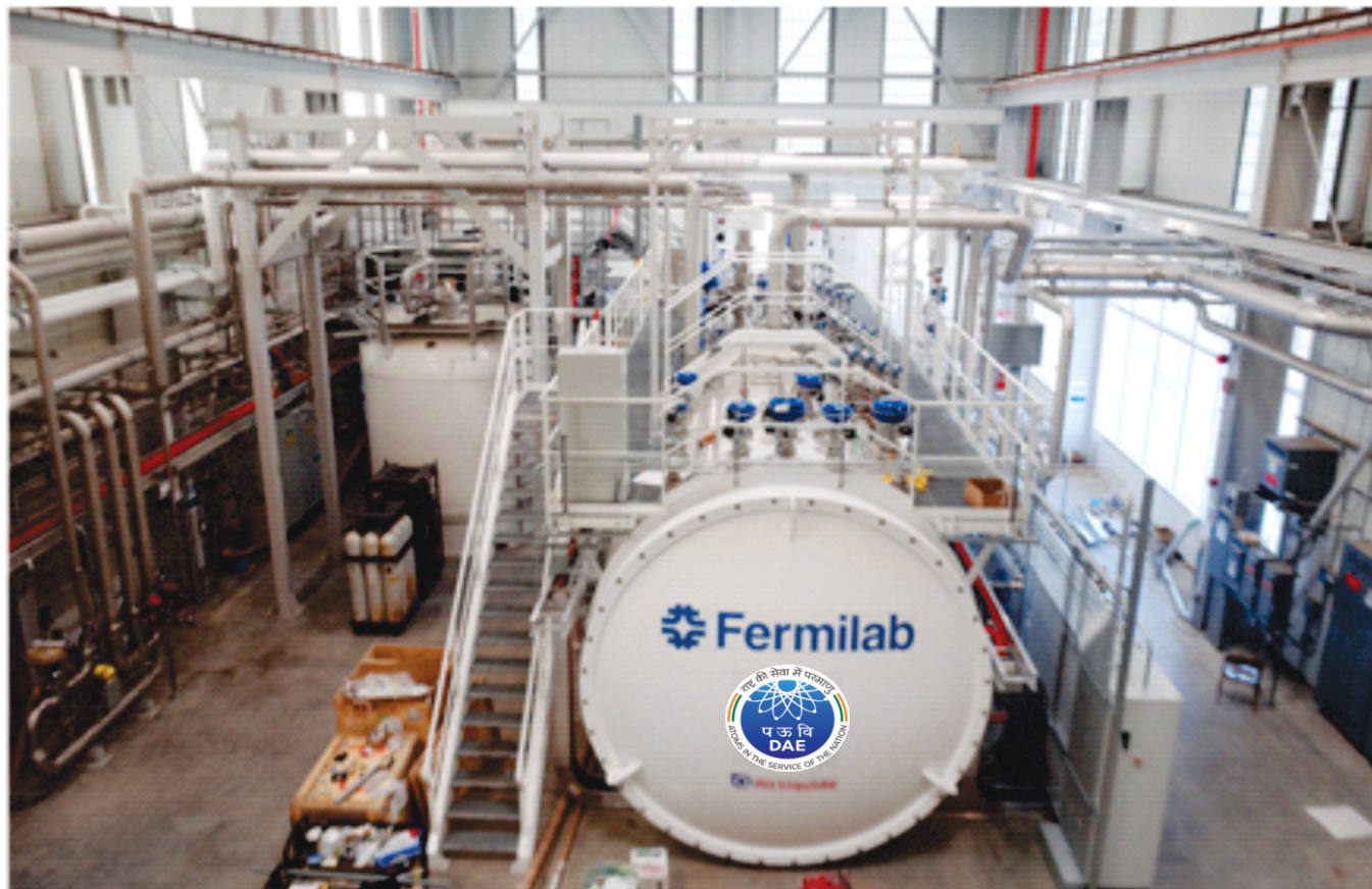
A 2 kW Cryoplant: Among important in-kind contributions of India to FNAL.
