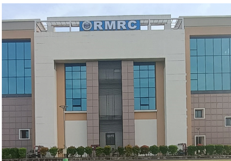
BARC's RMRC Facility in Kolkata.
