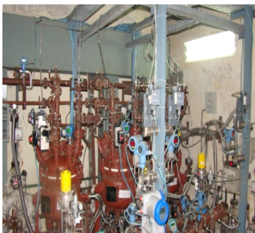
Fig.5: Feed system of Metallic Bunsen setup.
