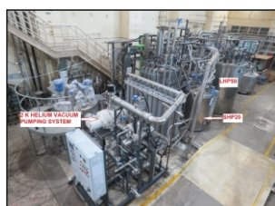
A view of the SHP20 cold box installation along with LHP50 cold box and warm pumping system
