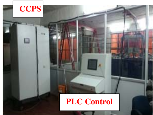
Fig.8 (a) Photograph of Capacitor bank charging power supply & PLC unit
