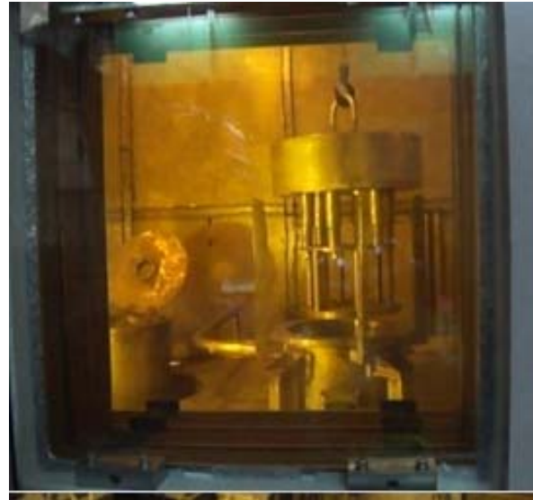
Filter / filter bag replacement
