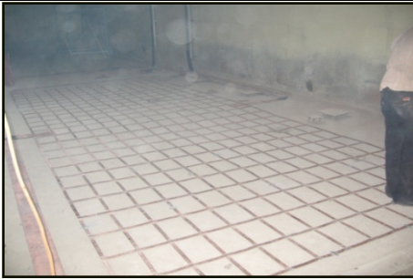
(a) RF grounding mesh at Klystron Gallery at CFB
