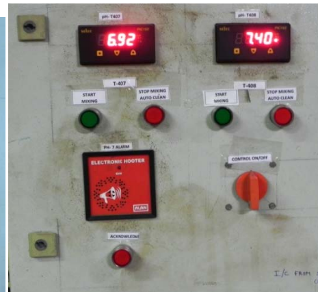
Figure 3: Power cum control panel
