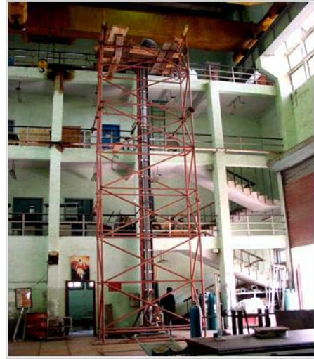
Fig. 3; Vertical set up for Tube Bundle for welding of tube to tube sheet
