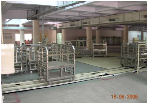
Fig. 8: View of Conveyor system outside the cell area
