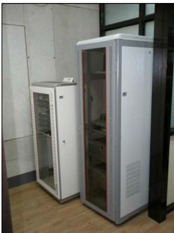
Fig. 3: IERMON Server Room
