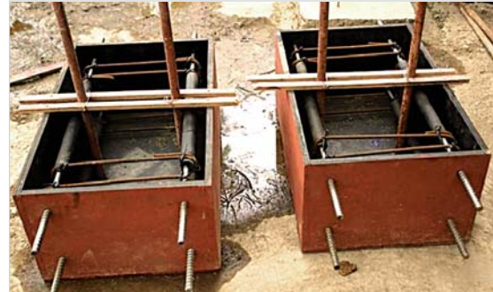
Fig. 3: Formwork of Specimen (CFB Site, A&CED, BARC)
