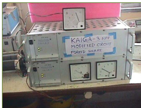
ECPS-II 100W & 60W testing for Kaiga-3/4 and RAPP 5/6 systems after development (2005-2007) at RCnD
