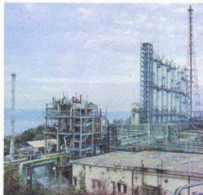
Fig. 1 BARC on-line fatigue monitoring system implemented at Heavy Water Plant, Kota
