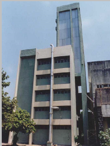
Integral Test Loop (ITL): A scaled test facility based on power to volume scaling for thermal hydraulic simulation of AHWRs
