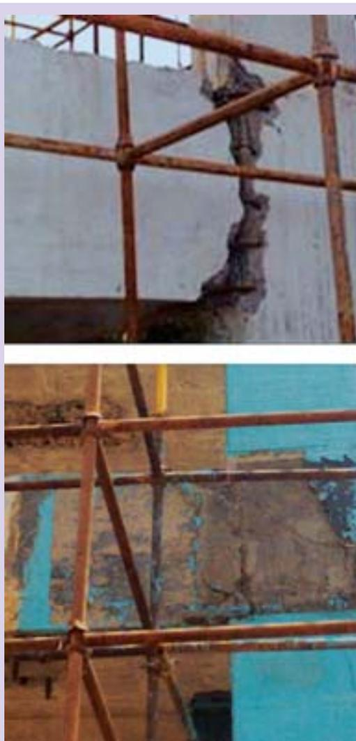
Fig. 6: Failure of beams of as built and retrofitted structure
