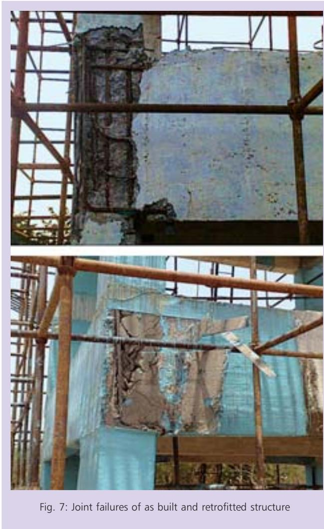
Fig. 7: Joint failures of as built and retrofitted structure
