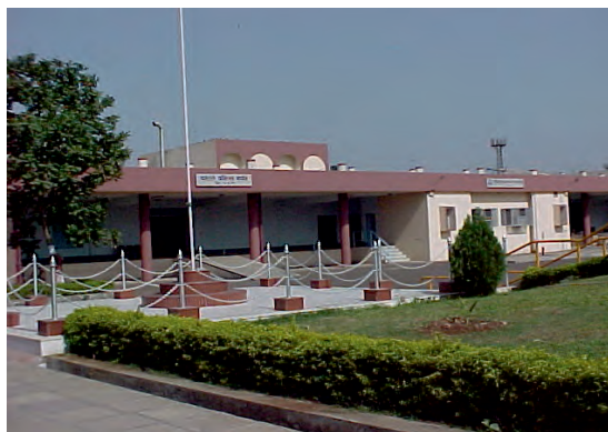
Figure 4A: Radiation Processing Plant, Vashi
