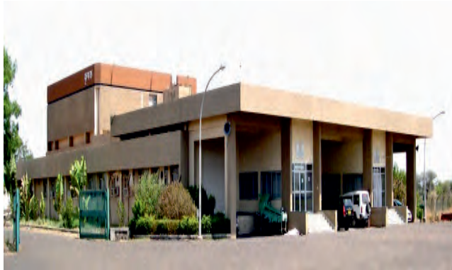
Figure 5: KRUSHAK Irradiator, Lasalgaon
