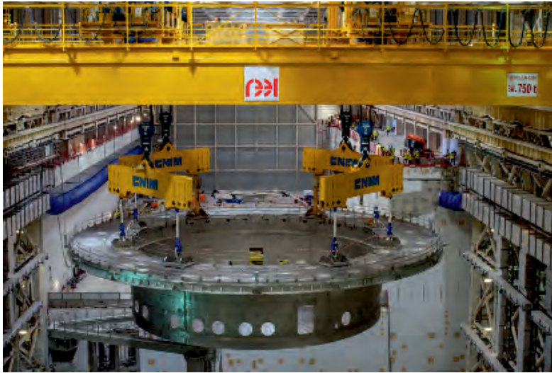
Figure 3: Cryostat base of ITER at ITER site, manufactured in INDIA
