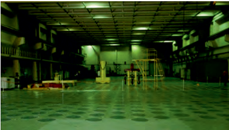
Solid Storage Surveillance Facility, Tarapur
