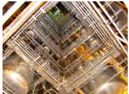
Inside view of hot cell of reprocessing plant KARP
