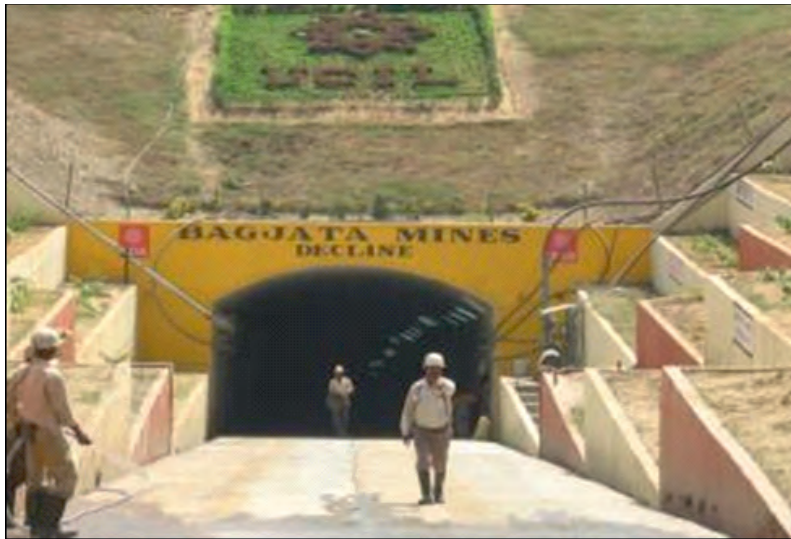
Fig.6: Decline Entry of Bagjata Mine
