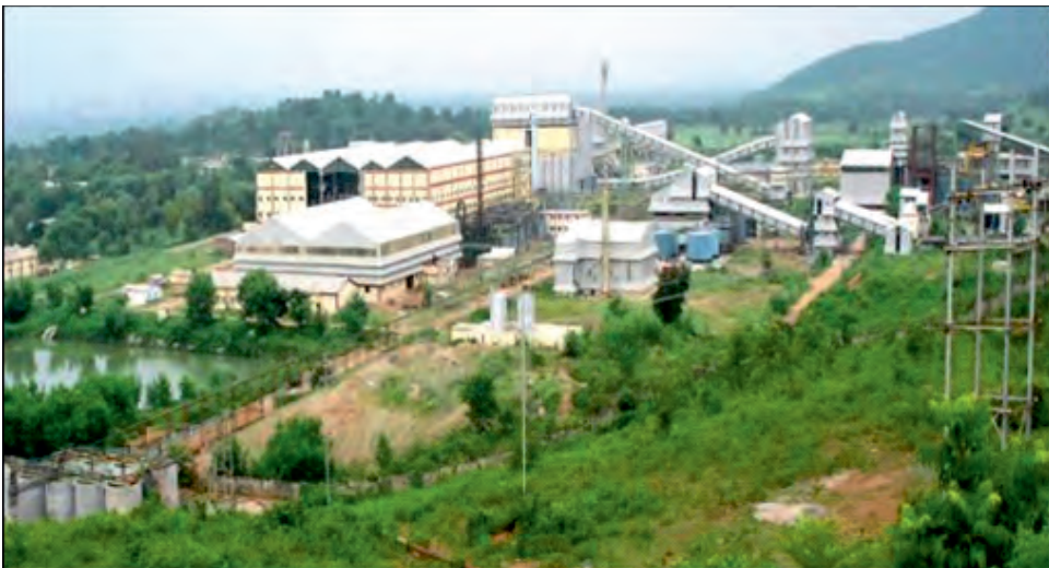
Fig.9: Aerial view of Turamdih Processing Plant
