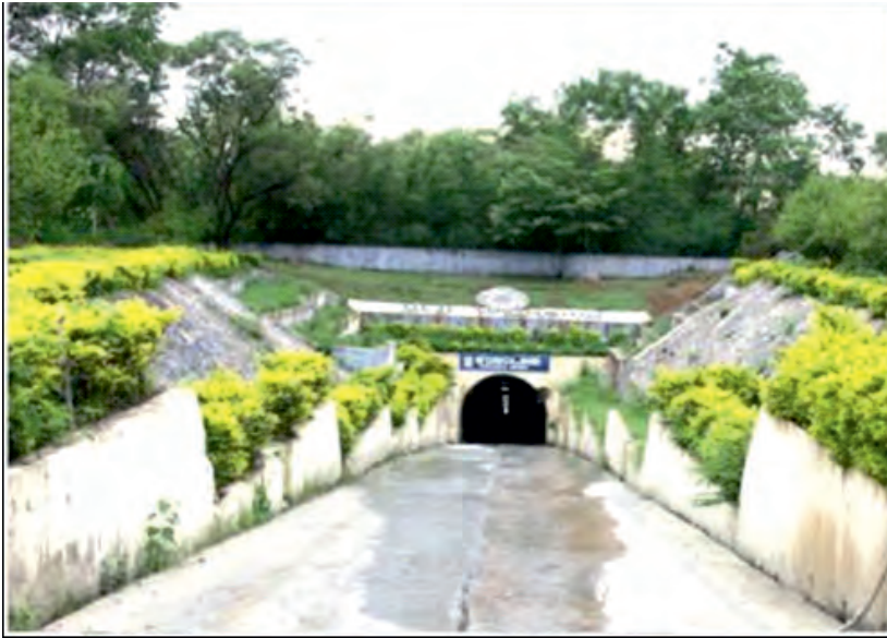
Fig.7: Decline Entry of Turamdih Mine
