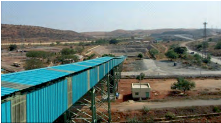
Fig.10: Decline Entry of Tummalapalle Uranium Mine
