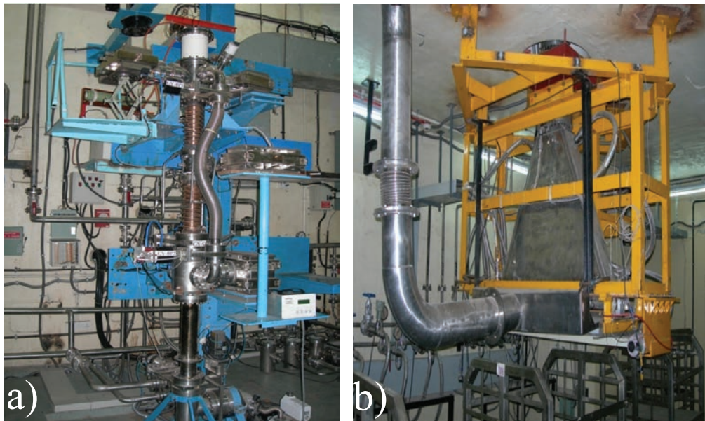
Figure 9.10: a) First Floor View of RF Linac, b) Ground Floor view of RF Linac.
