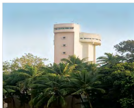
Fig. 13: 14 MV Pelletron + Superconducting LINAC
