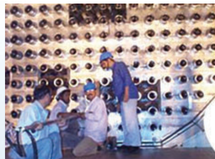
Visual inspection being carried out in TAPS 4
