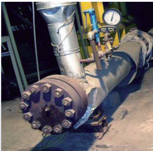
Fig. 2 : Fuel Locator Test Facility
