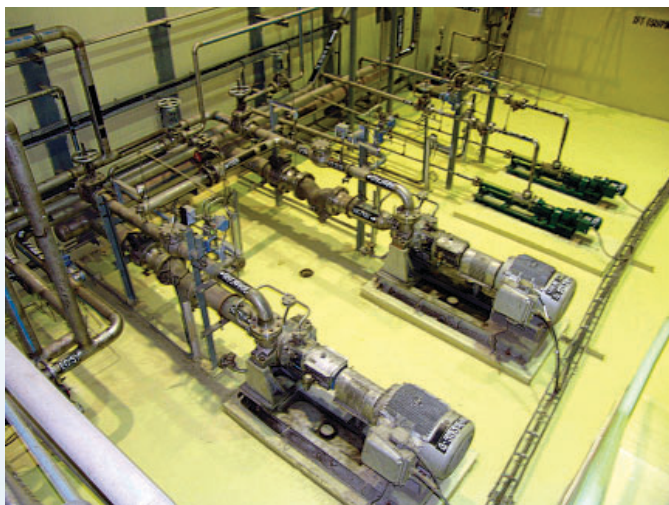
Fig. 5: Shuttle transport pump
