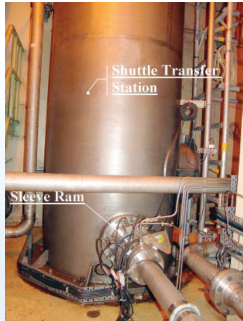
Fig. 4: Shuttle Transfer Station (STS)
