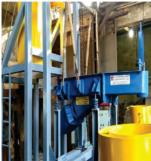
Fig.8: Remote handling of EMV Feeder
