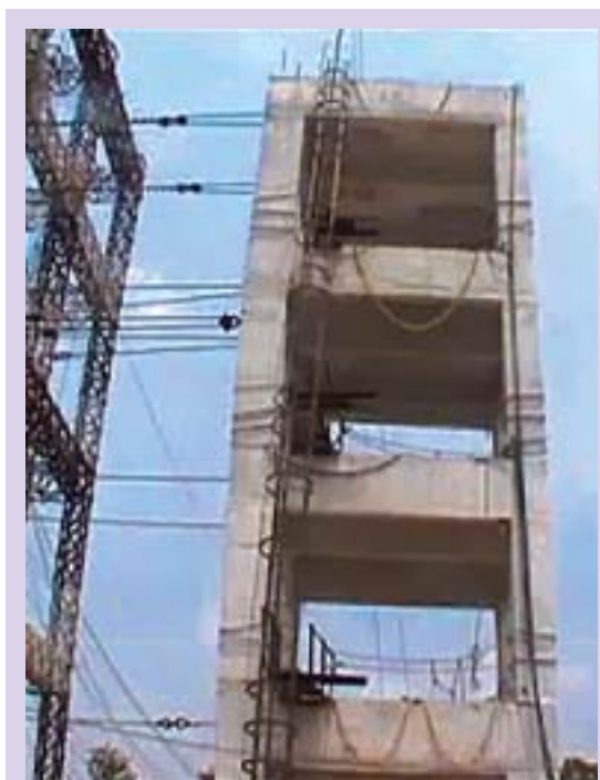
Fig. 1: Testing of original structure
