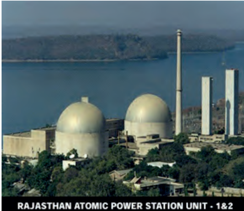
Fig. 3: Rajasthan Atomic Power Station 1&2
