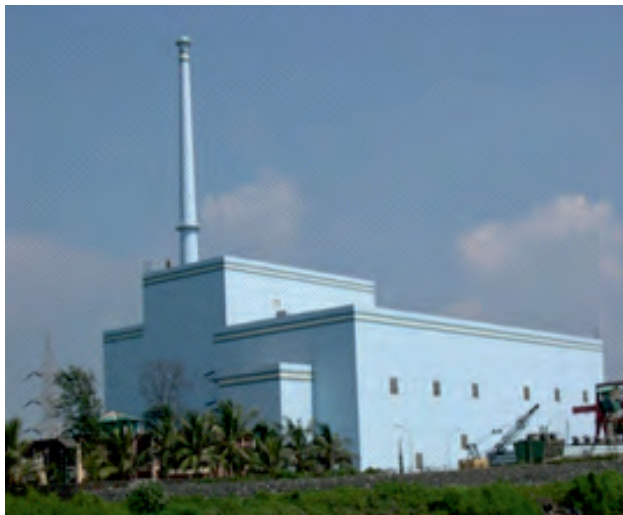
Fig. 2: Tarapur Atomic Power Station 1&2
