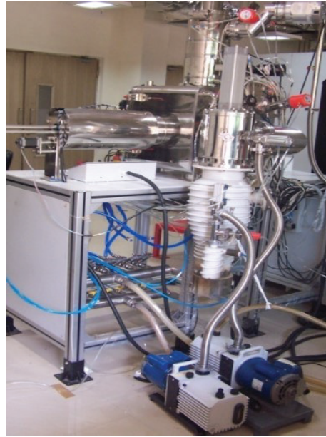
Figure 6.4: Photograph of Vacuum Plumbing Line for 10 kW System.
