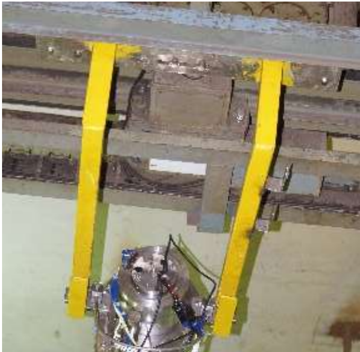
The System Installed on the In-cell Crane at Site
