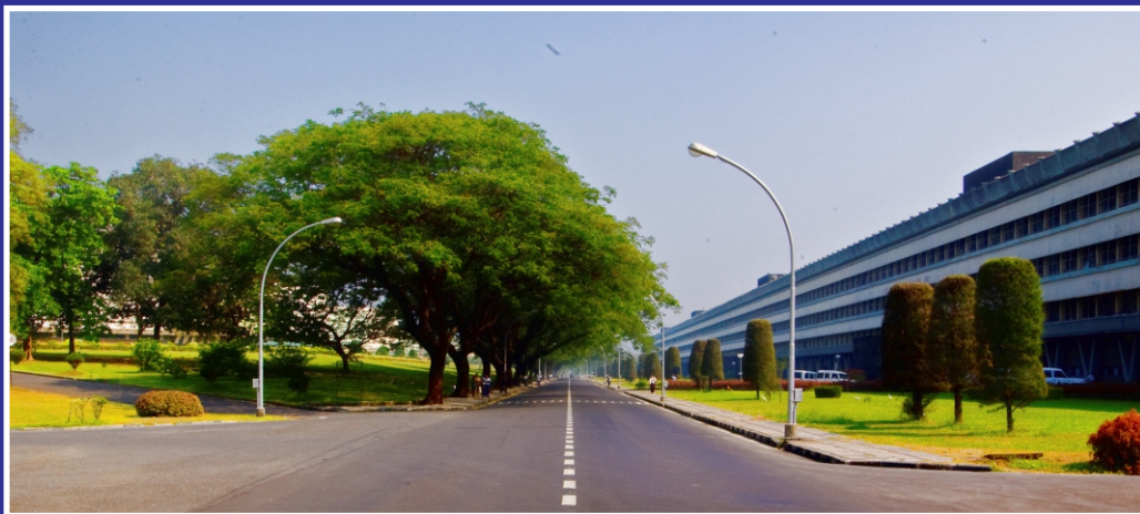
Modular Lab at BARC
