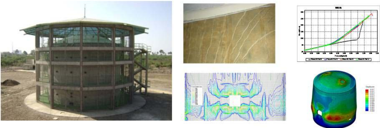
Fig. 7: BARCOM Test Model and Longitudinal & Shear Cracks around MAL & Embedded Sensor Response during Over-Pressure Tests on July 23-24, 2011 (1.78 Pd) & Oct 02 2011 (1.68 Pd) and Numerical Simulation Results
