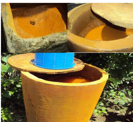
Fig. 4: Existing filtration systems for remediation of iron at Monojili village, Tejpur, Assam
