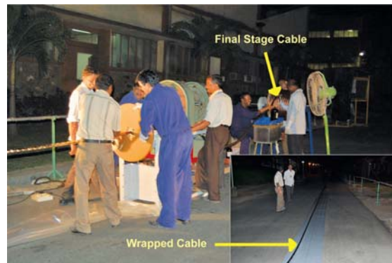
Fig. 8: Foil wrapping on final stage cable
