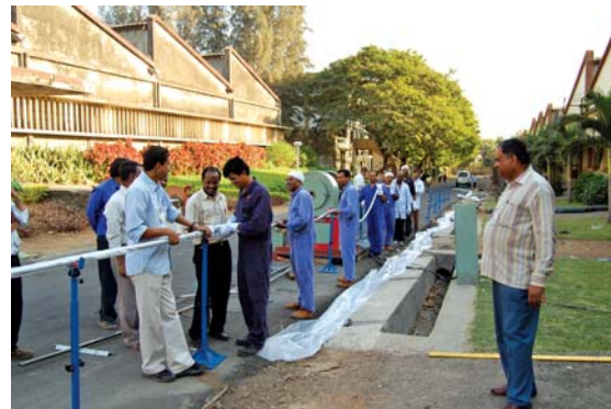
Fig. 9: Insertion of wrapped cable in circular tube
